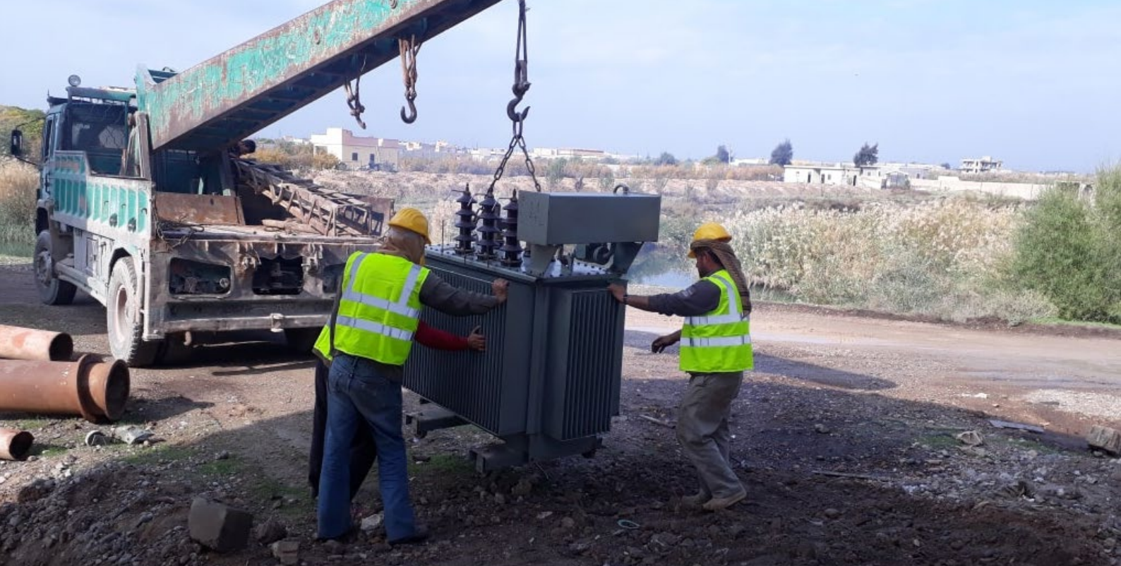
Figure 9.2: Installation of new transformers by the RCC
